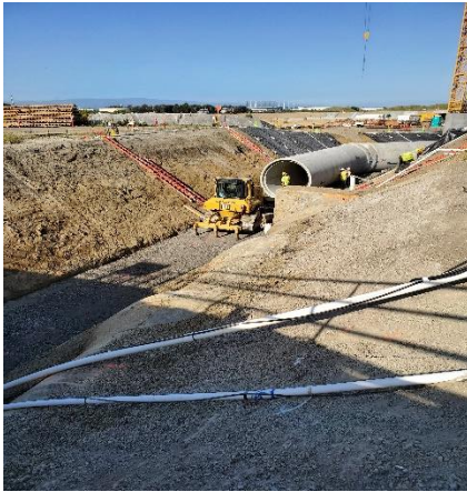
Underground work 96" and 108" exposed
